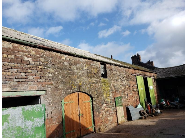
Potential barn roofs for solar modules
