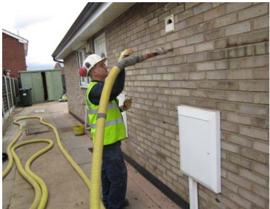
Wall Cavity Insulation. Photo credit. Yes Energy Solutions
