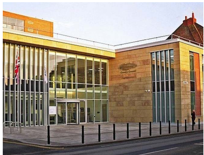
Cumbria County Council building in Carlisle. Photo credit: Rose and Trev Clough/ Geograph
