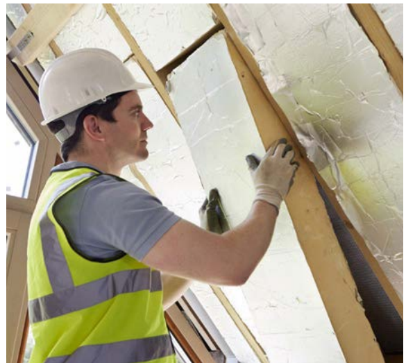
Installing insulation boards. Photo credit: edie newsroom
