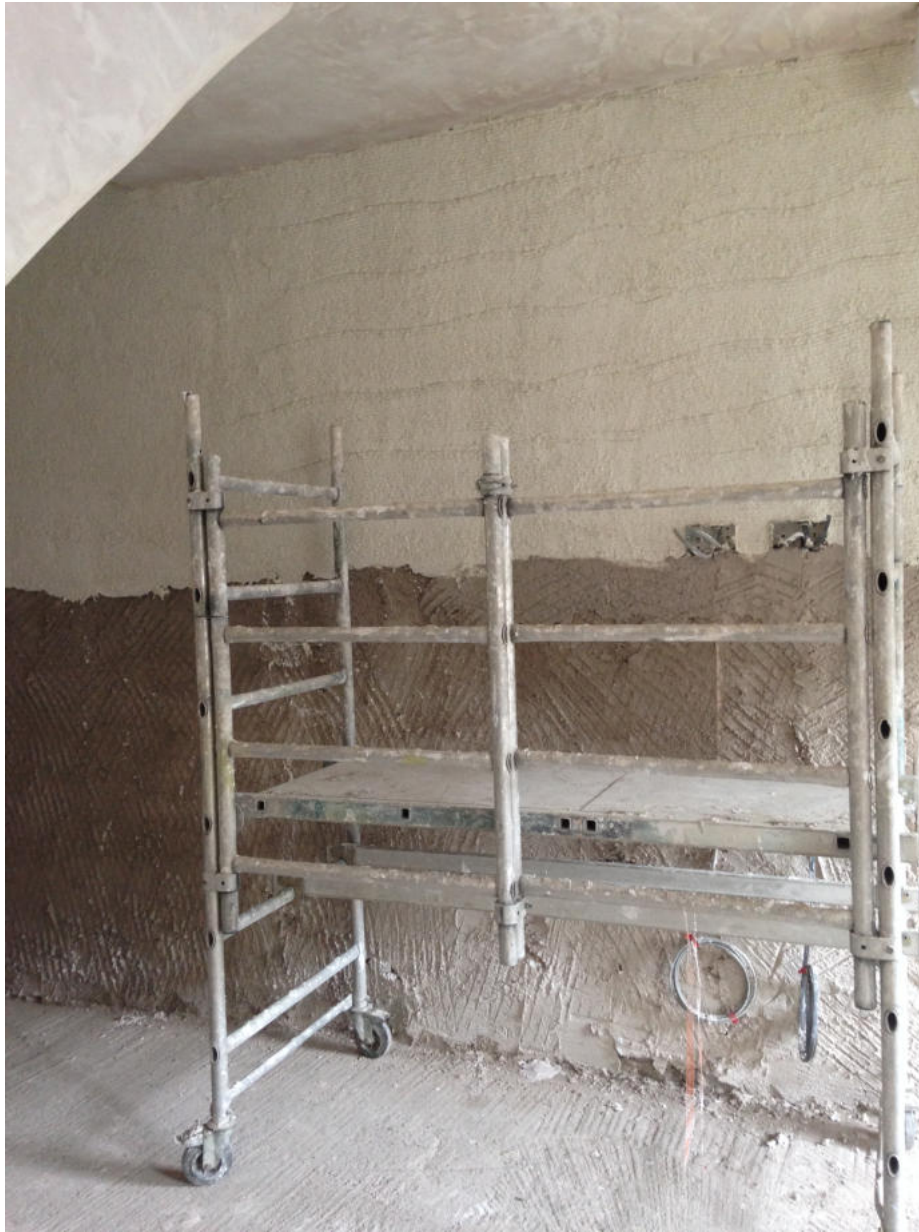
Soild ground floor – limecrete U-value 0.23W/m2K
