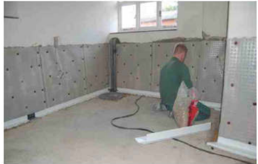
Newton 508 Mesh and Basedrain installation
