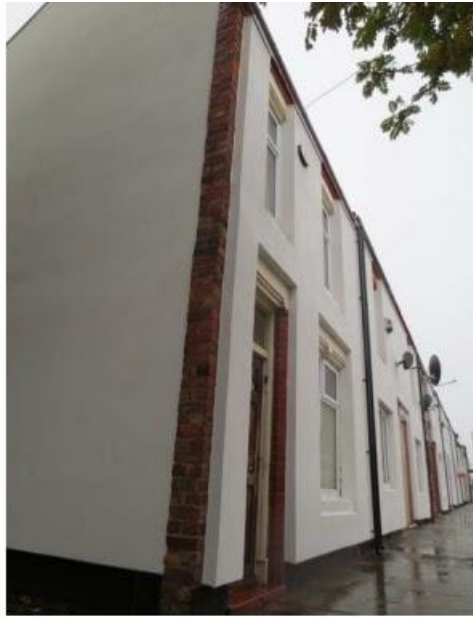
Figure 24 Note large areas of exposed building elements
