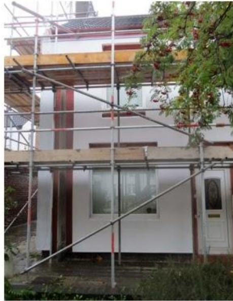
Figure 25 Large thermal bridge created by lamppost
