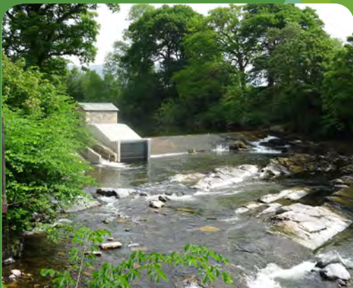
The turbine house, screw housing and fish pass
