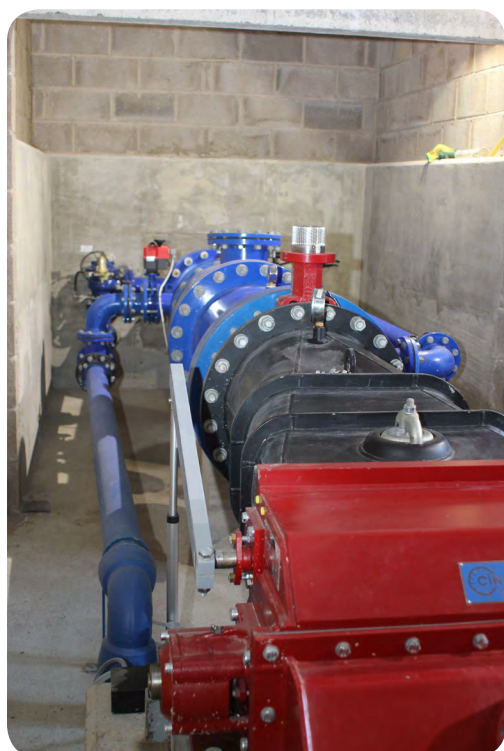
The new hydro turbine installed and commissioned
