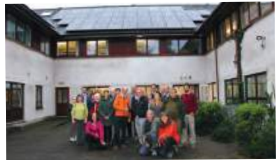
Community-owned solar panels at the Lake District National Park Authority
