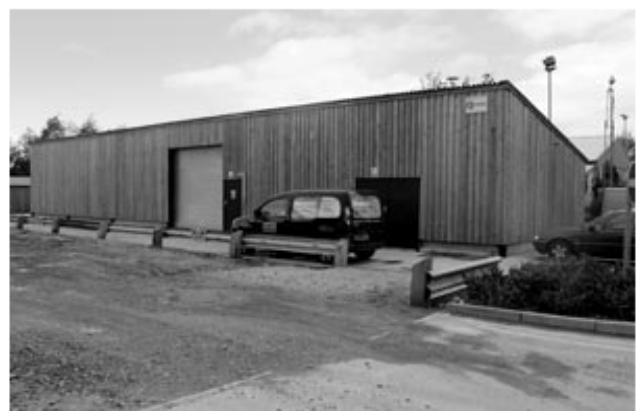
Biomass Energy Centre Building and fuel store
